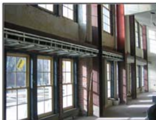
The new library will include the original west facade wall
