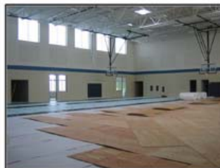
The new, larger gym features large window for abundant natural light
