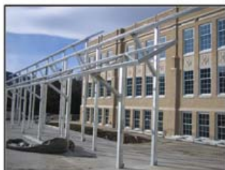
Solar panels will be mounted on the south side of the school and will provide shade for bicycle parking
